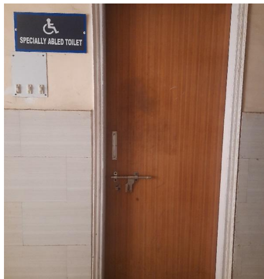
Figure 6. Disabled-friendly washrooms with signage
