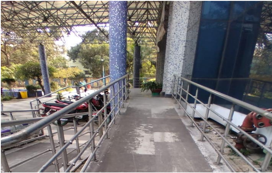
Figure 3. Ramps for Easy access to the University buildings
