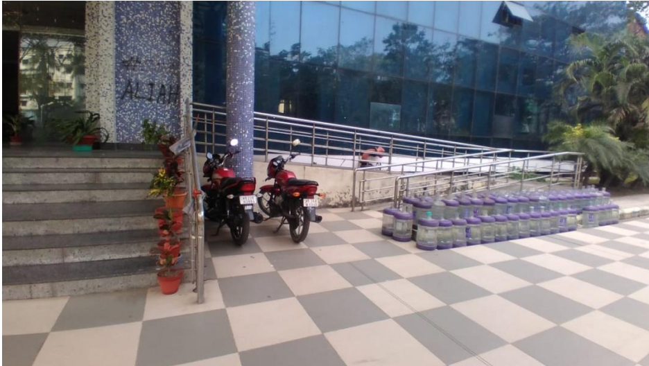
Figure 1. Ramps for Easy access to the University buildings
