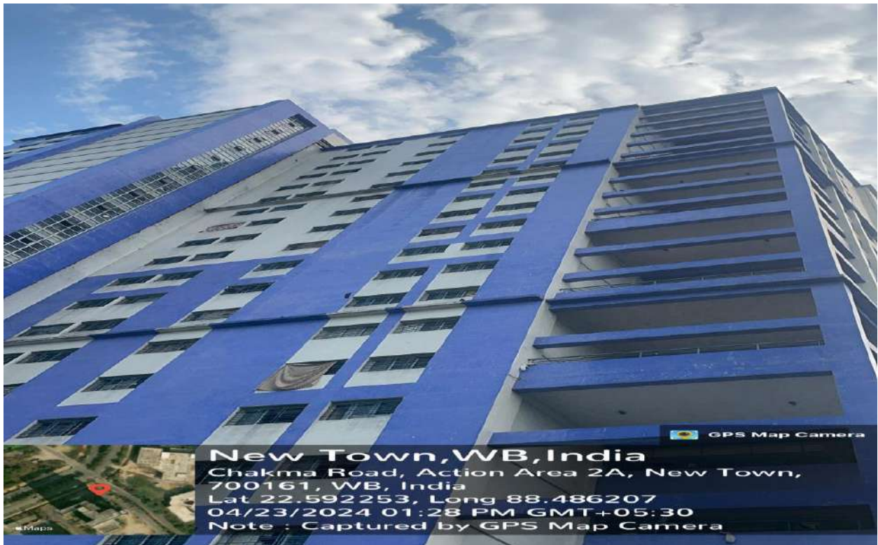
Figure 12: Hostel at the Main Campus
