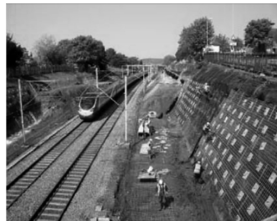
Figure 23.38 Soil nailing for railway. (After Prashant and Mukharjee, 2010)
