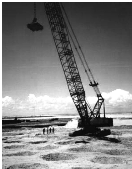
Figure 23.6 Dynamic compaction.
