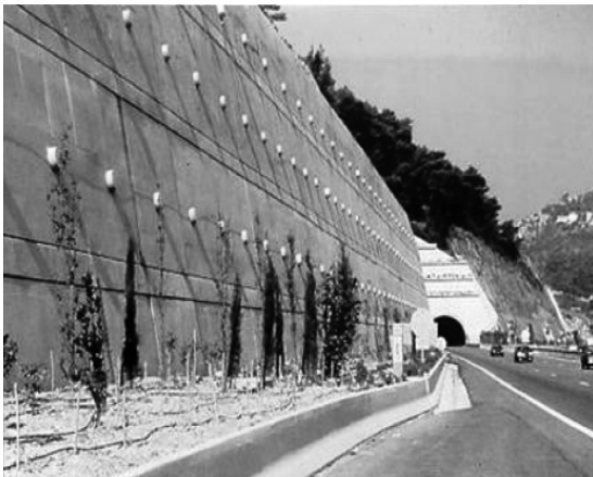
Figure 23.37 Soil nailing for highway. (After Prashant and Mukharjee, 2010)
