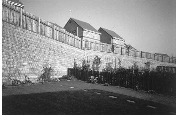
Figure 23.26 Finished view of a reinforced earth wall with differential grade.
